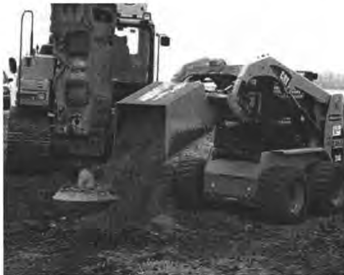
Figure 5.5. High-energy, low-frequency hammer used for the construction of Geopier foundations.
